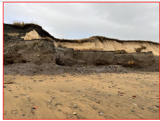
Accelerated erosion of the softer sand mantled on the colliery spoil platform (/3401C01)
