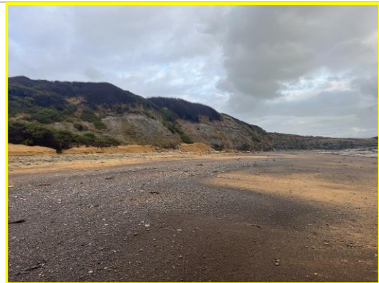
Localised rock falls in harder cliffs to the north. Clinging in the finer beach material in foreground (/3301C02)
