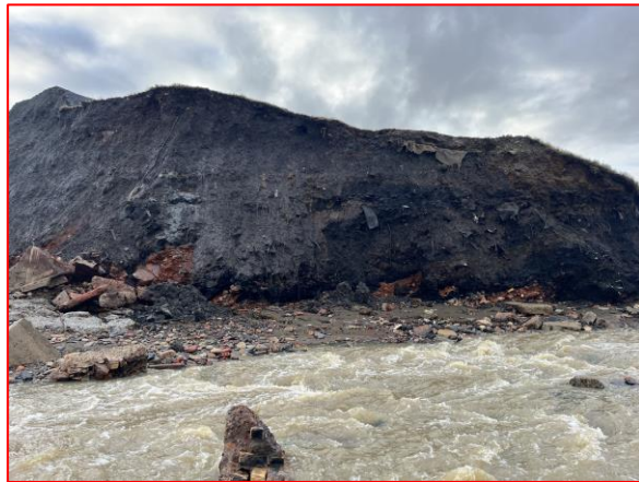
Erosion of backing man-made cliffs at the mouth of the river Lyne (/3401C06)
