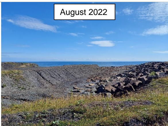
North Rock Revetment end and outfall channel (/3401C07)
