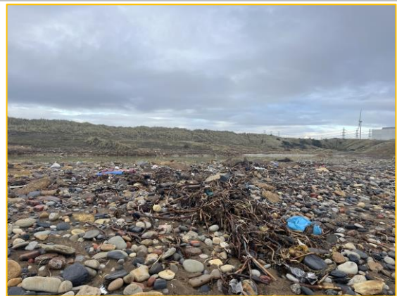
Significant storm deposits along colliery spoil platform (3501/C01)
