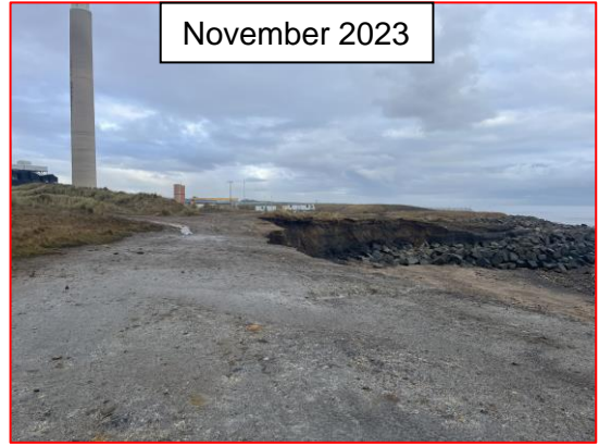
Eroding cliff to the north in November 2023 (3501/C01)
