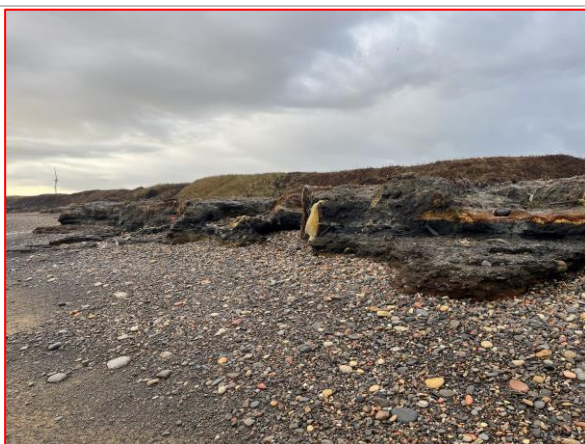
Eroding colliery spoil platform (/3401C01)
