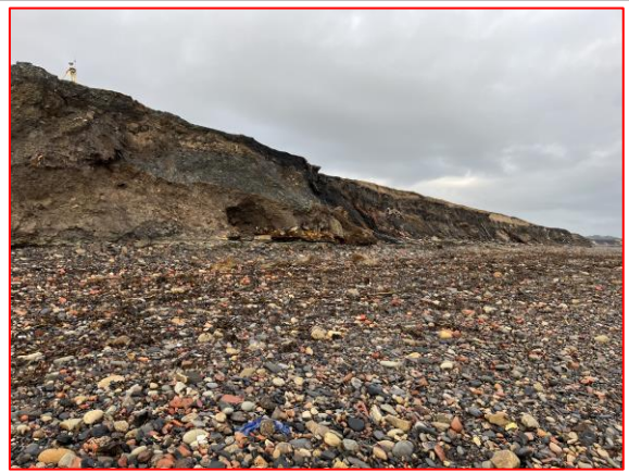
Erosion of backing man-made cliffs, releasing colliery spoil and refuse to the foreshore (/3401C05)
