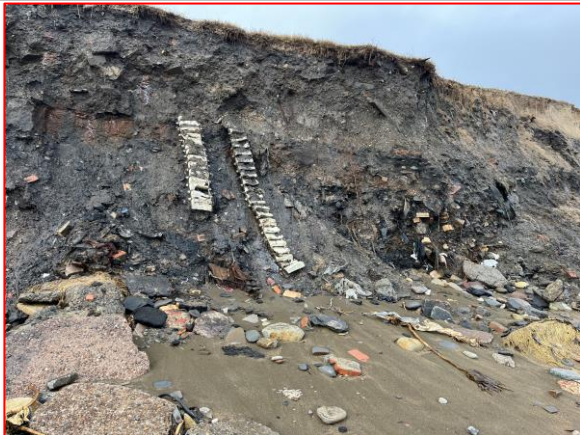
Erosion of backing man-made cliffs, releasing colliery spoil and refuse to the foreshore (/3401C05)
