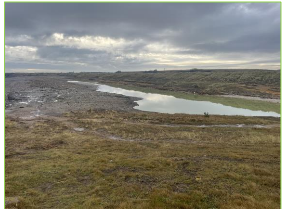
Water accumulation between the spoil's berm and the rear soft natural dunes (3501/C01)
